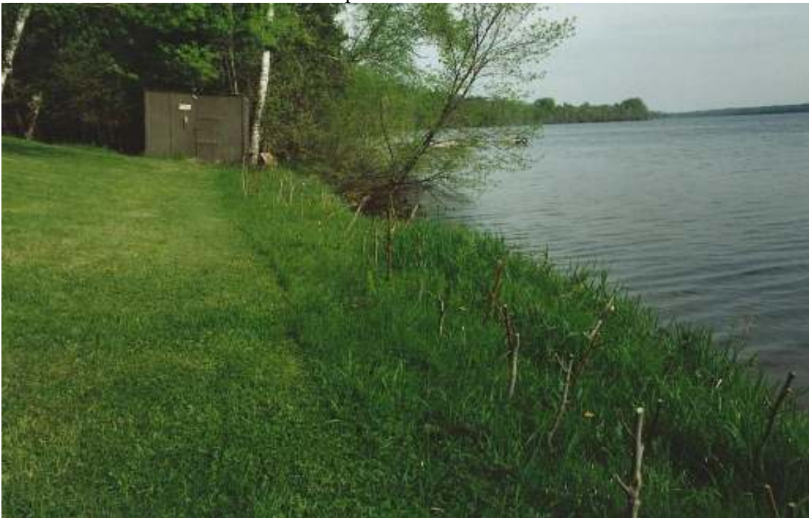
Photo #6 – View of shoreline bank at the start of the planting willow and other bushes.
